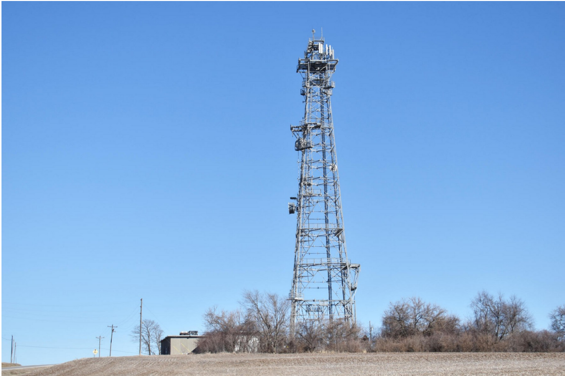
Tower seen from the west on Hitt School Road.
